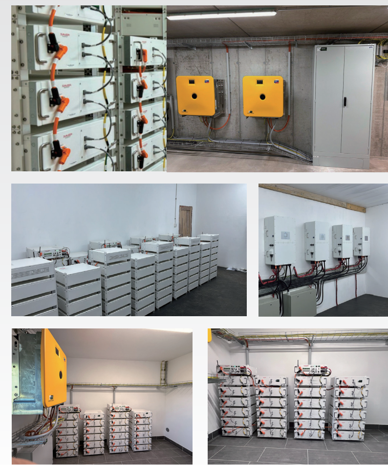
Austria OASIS Flex & SMA 100kW/480kWh Rack-mounted Battery System BESS for Commercial Building
