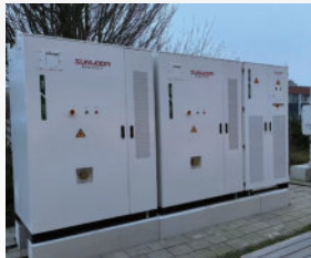
Netherlands OASIS L215 & Power 200kW/430kWh Outdoor Battery Cabinet System
